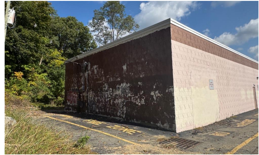
Rear of building, facing west.
