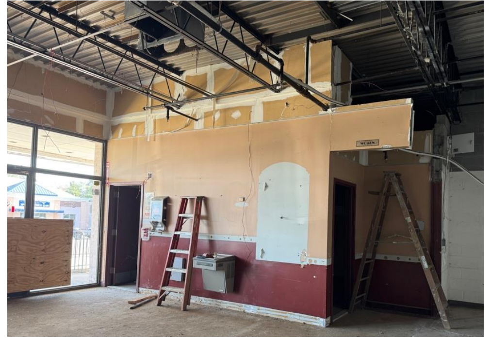
Above: Building interior in a state of vacancy.
